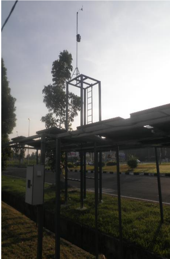
Figure 1. Weather station and PV array
