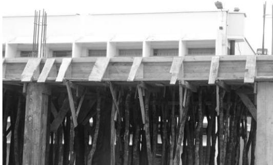
Figure 1 A construction site in Dar es Salaam using softwood formworks
