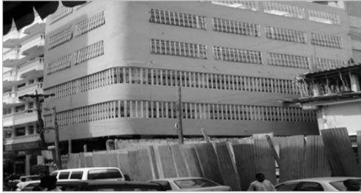
Figure 13 A building with metal grills on openings
