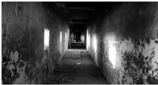
Figure 9 Windows without adequate fire resistance in a wall.
