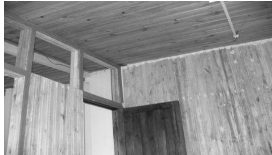
Figure 7 Timber partitions in an office building
